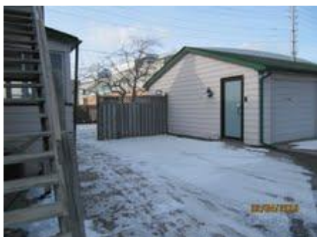
Entrance of the Admin Office
