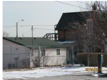
View of the Admin Office from Charles Street.
